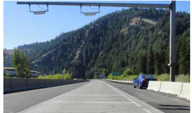
La Grande, Oregon WIM Site in I-84 Mainline
