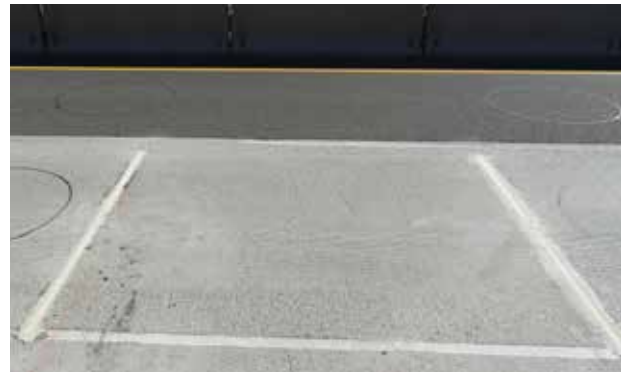
Four WIM sensors are installed in two pairs in traffic lane
